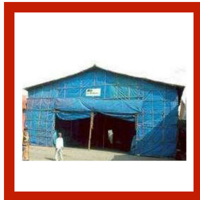
FRP Coated Monsoon Shed on Rent
